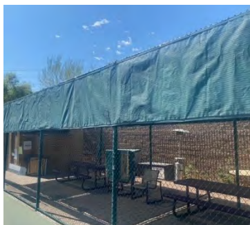
Maintaining Shade structures Replacing all the tie-downs on shade
